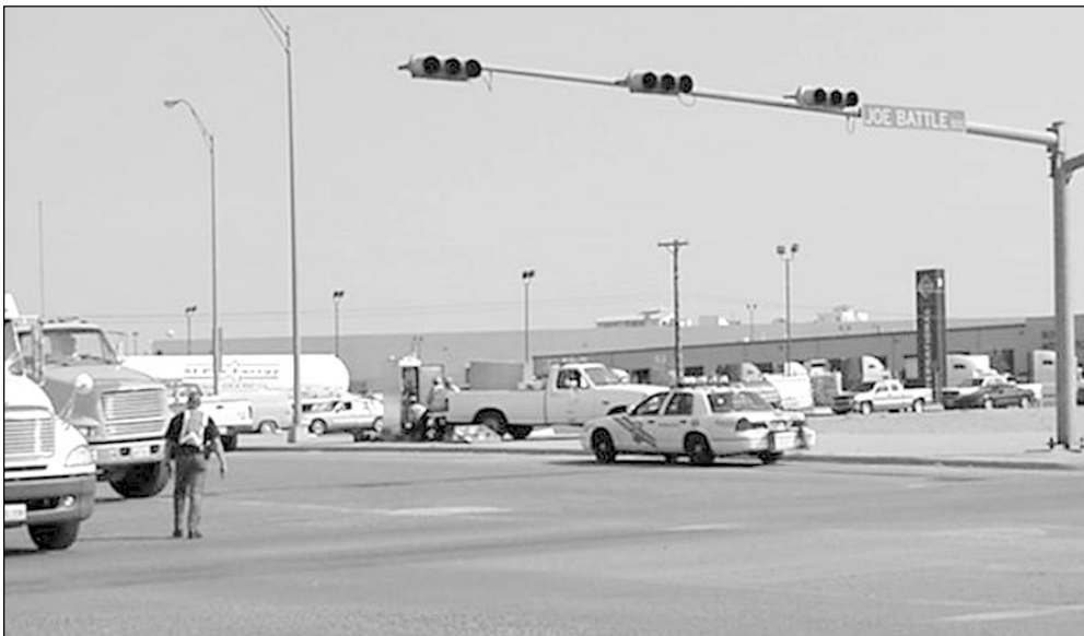
GIVING DIRECTION — Monday's rain storm caused malfunctioning in the traffic signal at Joe Battle and Rojas. El Paso Police were providing manual assistance Tuesday morning as crews worked on the mechanism.
