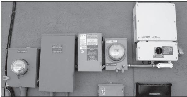
PRESTO CHANGO - The solar panels capture the energy from the sun and transmit it to an inverter system, shown above. The inverter system transforms direct current (DC) into alternating current (AC) and then sends it into the breaker box that distributes the electricity into the home.
