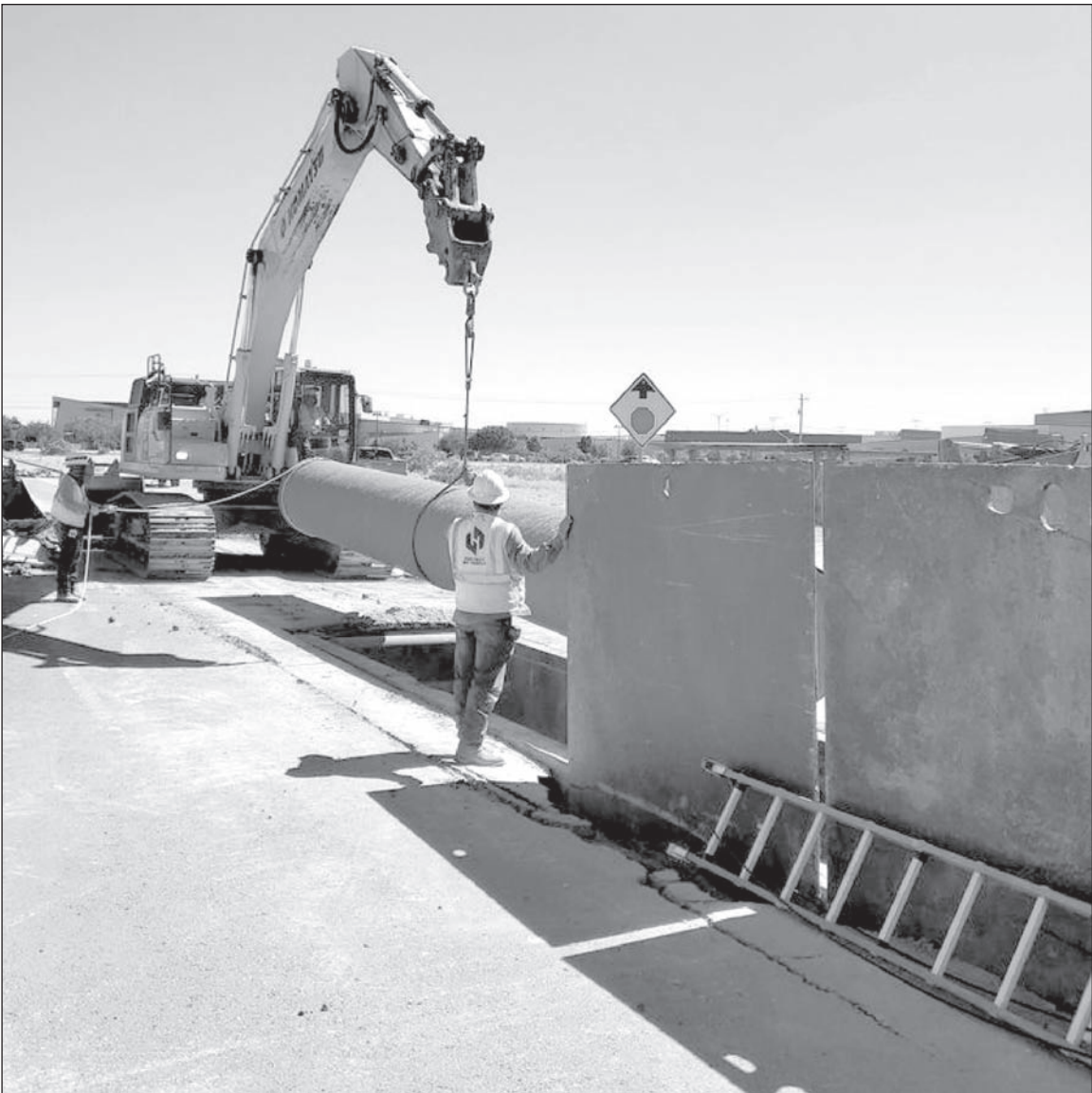
BIG PIPE – Crews install the 36-inch line along John Hayes.
