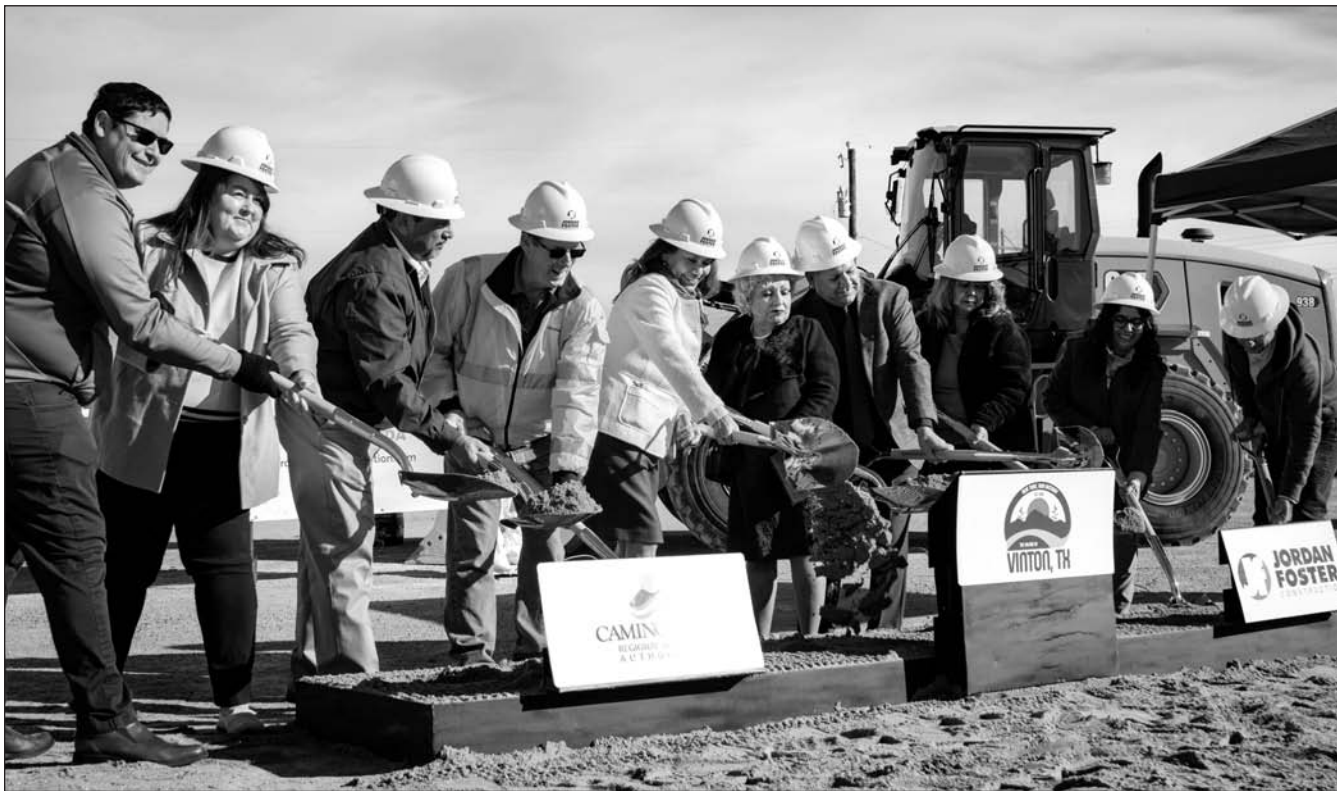
GETTING BUSY – The recent groundbreaking by Village of Vinton officials marked the start of construction on the Valley Chile Road infrastructure project. Community members, government officials, and media representatives joined Village officials for the event.
