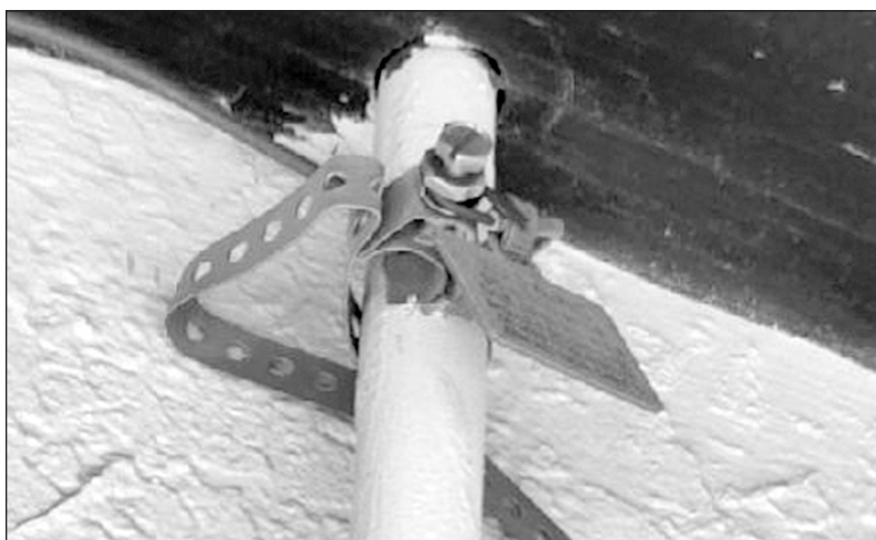
JUST WAITING TO HAPPEN – The loose ground strap, above, is literally being held off of the bare metal by the retaining screw. Paint covering the conduit around the backside keeps the strap off of bare metal.
